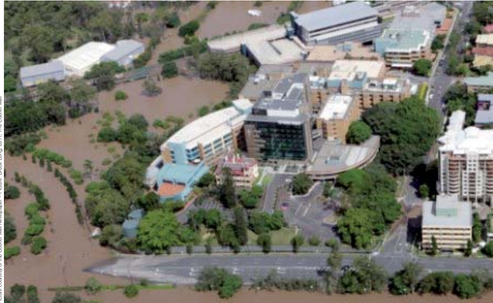
The Wesley Hospital (Brisbane) surrounded by flood waters
