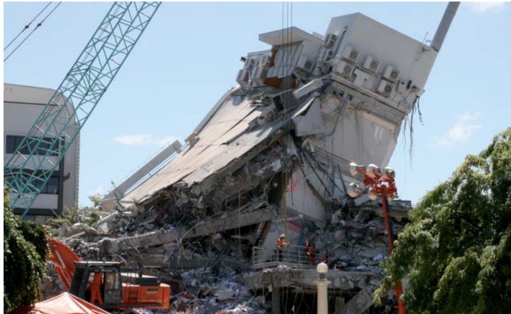
Pyne Gould Building after Christchurch earthquake
